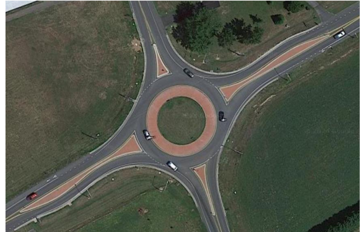
SR 10 @ SR 15, Roundabout
