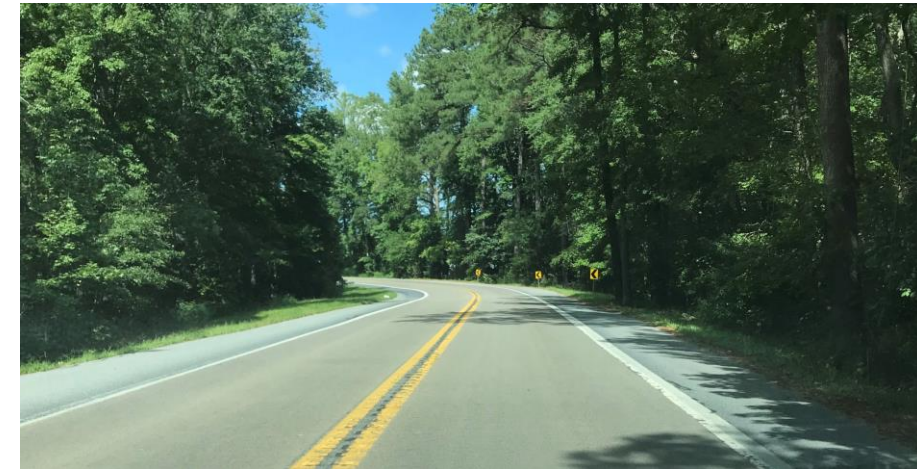
High-Friction Surface Treatment – Gravel Hill Road
