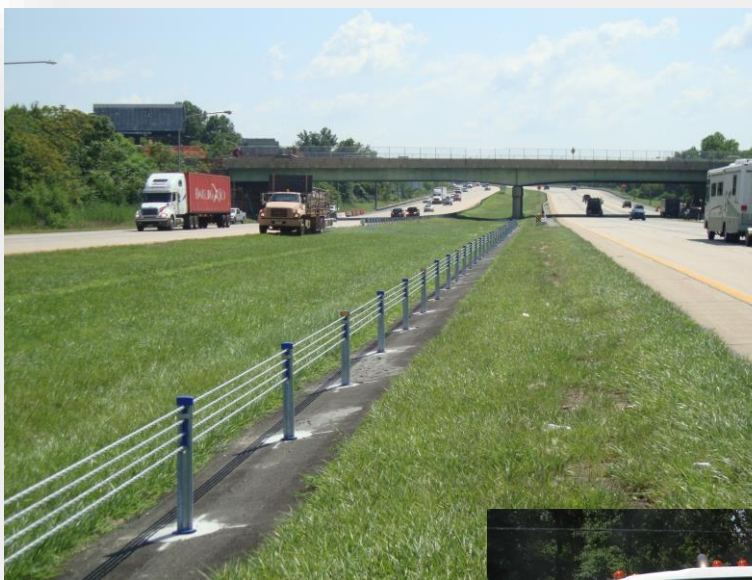
High-Tension Cable Barrier
